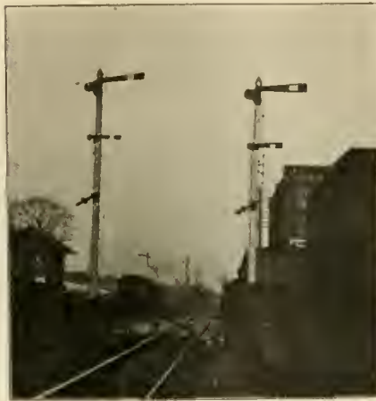
AUTOMATIC SIGNALS, LOWER AND SHORTER ARMS INDICATING THE DIVERGING ROUTE.
